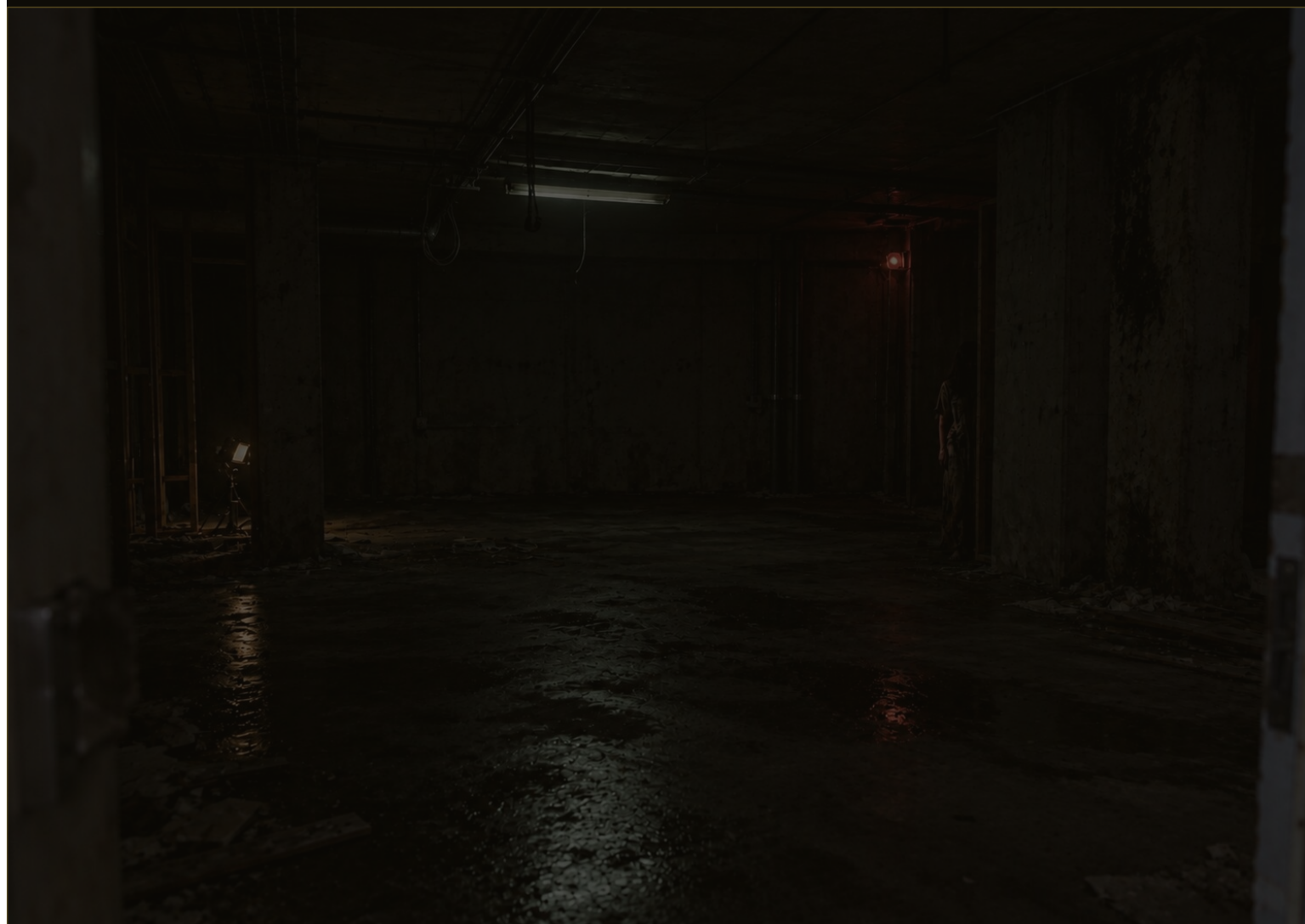
Wing C — the flooded lower corridor.
